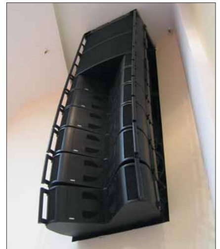
An Outline Butterfly array installed in the main hall of the DK Neftyanik centre in Uray
